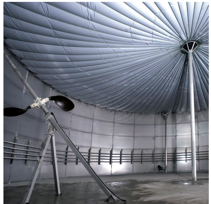
Figure 7 Inside view of a stainless steel biodigester, showing the agitator mechanism on the left hand side
